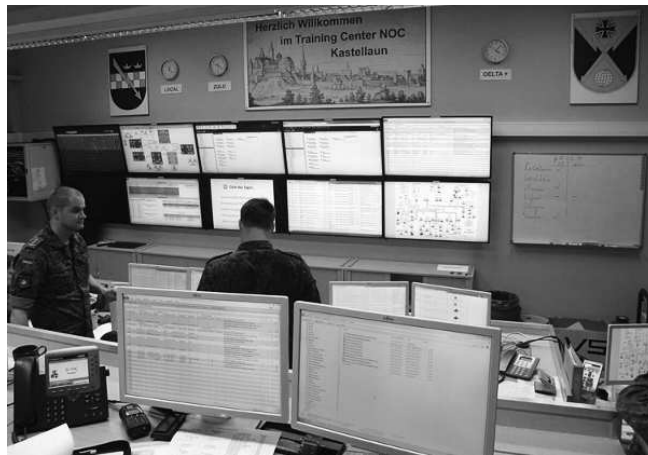
Das Network Operation Center (NOC)
